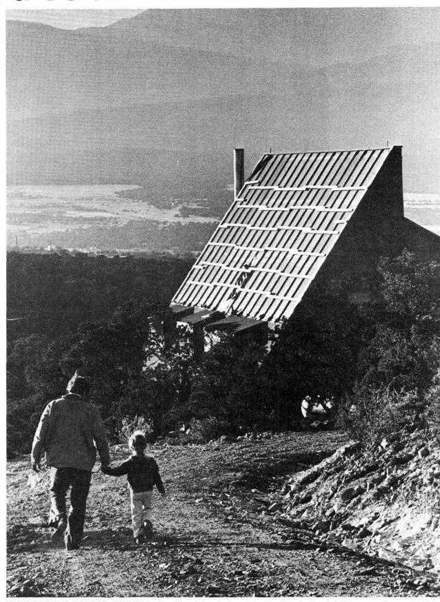
HOUSE LOOKS ACROSS VALLEY to Sandias rising in the distance. The horizontal braces on the roof will be removed as transparent sheets are installed.
